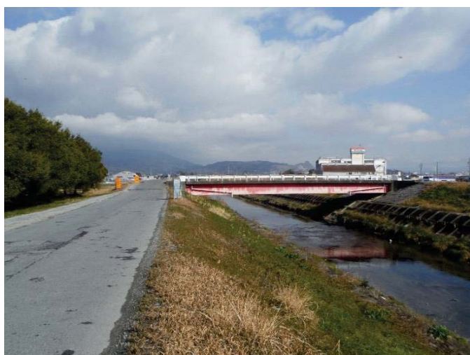
菰田橋着工前
